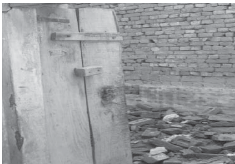
Inside view of a semi-constructed house
