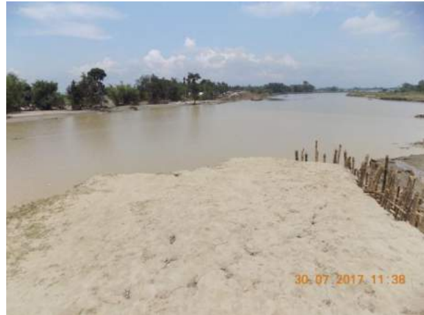
The Ranganadi&Spot of the breach of embankment in Jainpur area
