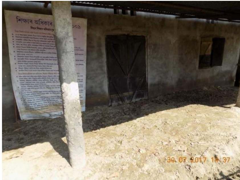
Silt deposited at the door of a classroom in the primary school at Majgaon
