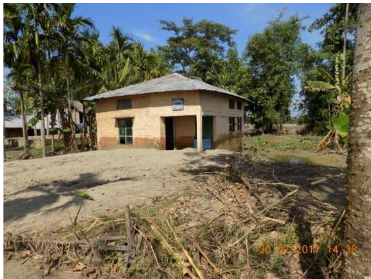
Silt deposited in and around the local Anganwadi at Majgaon
