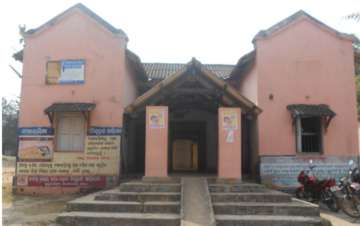
Maternity / Surgical Building, Dampara CHC
