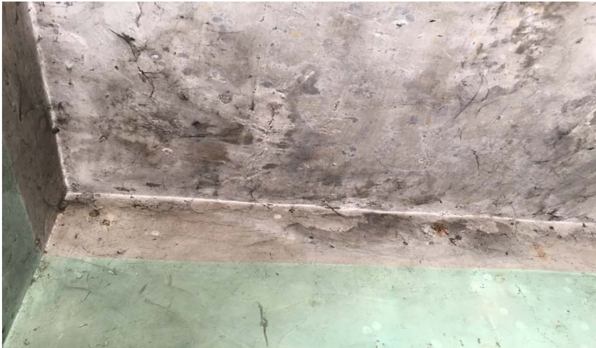
Smoke from the makeshift stove has blackened the ceiling and walls inside the AWC
