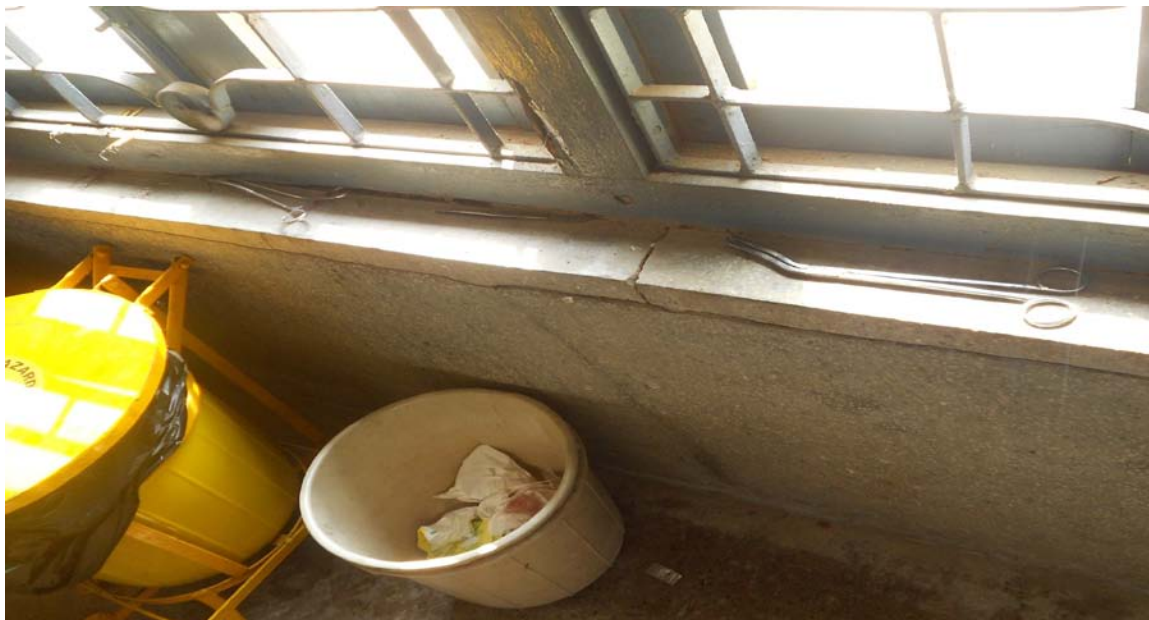
Medical instruments left on windows and biowaste in a garbage bins next to the proper disposal bins.
