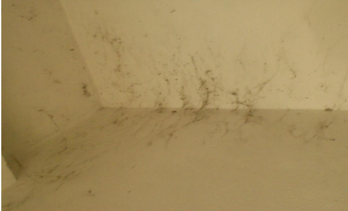
Ceiling above the AWC/VHND room
