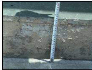
Entry into the Langar room (Kitchen) Absence of a ramp; flight of two steps with a total height of 9.5" (Mandoli Jail)
