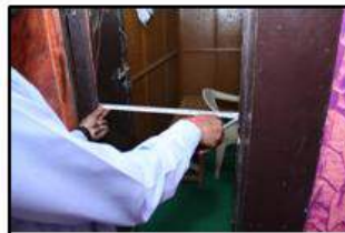
Entrance to the FM Room with a width of 18" (Tihar Jail)
