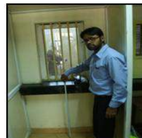
All 34 counters inside the Mulaqaat Room were at an appropriate height of 36". (Mandoli Jail)
