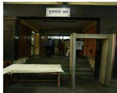
Flight of five steps with a total height of 28" leading to the Medical Inspection Room and Meeting Room (Rohini Jail)
