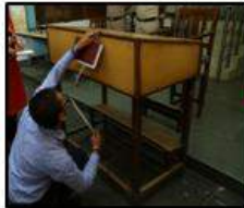
Registration table at a height of 48", inaccessible to a wheelchair user (Rohini Jail)
