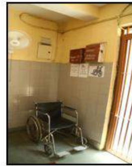
Presence of a wheelchair with signage upon entry into the building. (Mandoli Jail)
