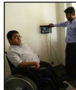
Upon entry into the Jail HQ, Biometric device placed at a height of 47" (Mandoli Jail)
