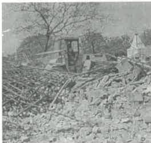
Concrete houses bulldozed at Bellilious Park
